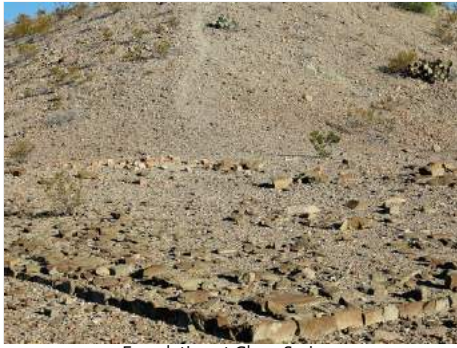
Foundation at Glenn Springs
